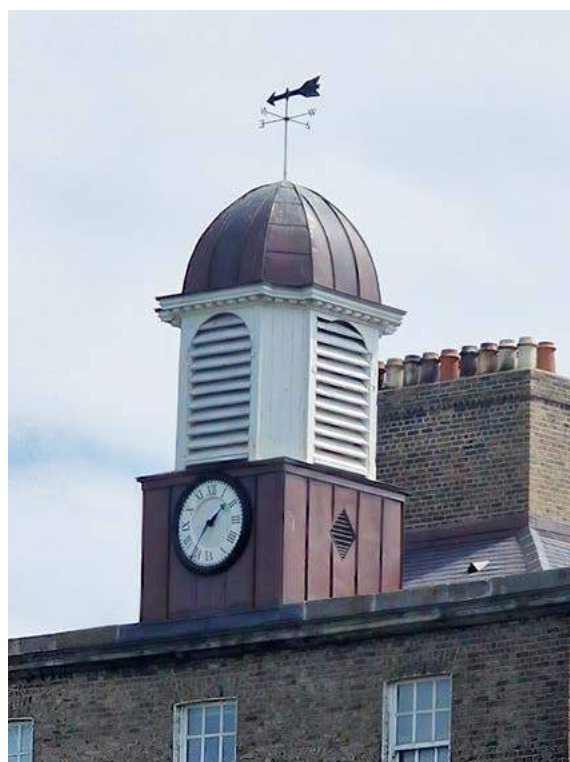
Figure 60: Copper-covered dome over louvred timber vent
