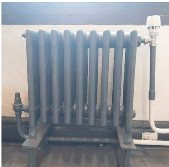
Figure 23: Cast-iron radiator with a thermostatic control
