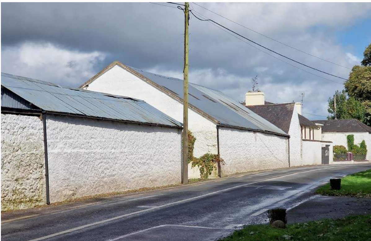
Figure 12: Limewash on traditional farm buildings
