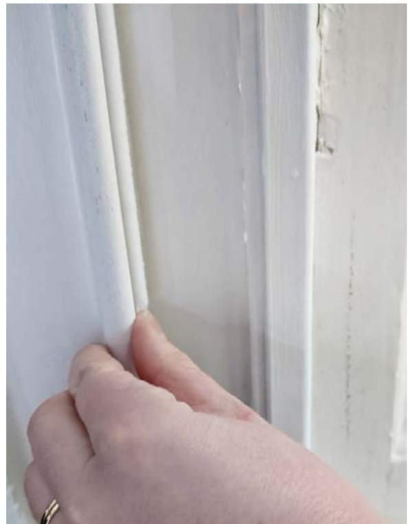
Figure 49: Discreet draught-proofing brush on a historic window
