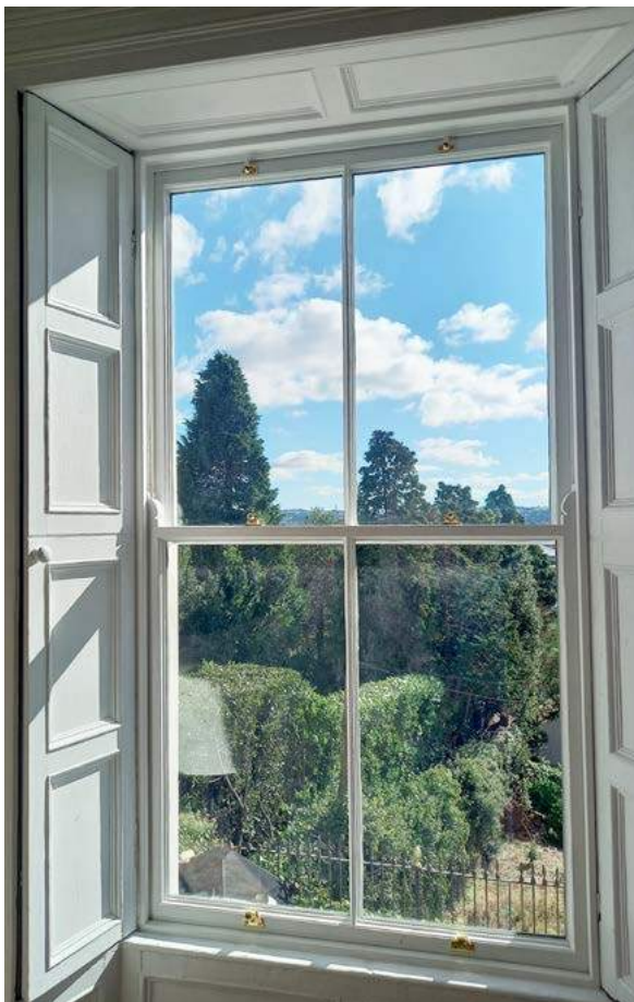
Figure 45: Two-over-two pane timber sash window
