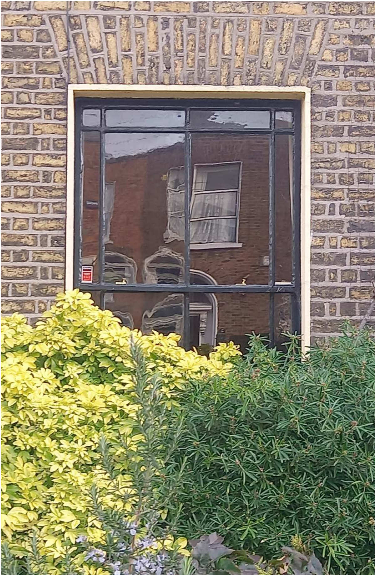
Figure 44: Timber sash window with original glass panes
