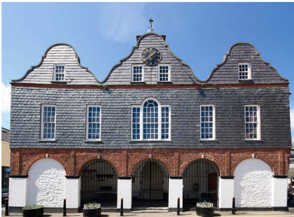
Figure 26: Natural slate hung front elevation
